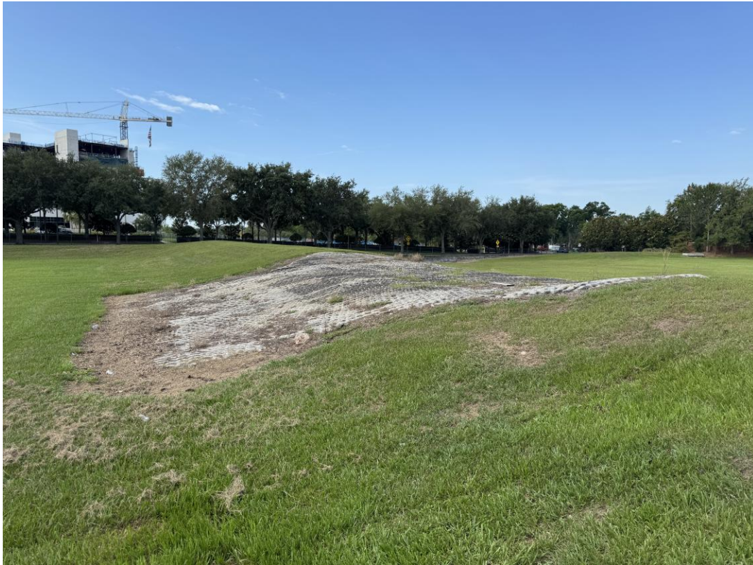
PHOTO #8.2 – Stabilized spillway from A1 West to A2 on May 23, 2025
