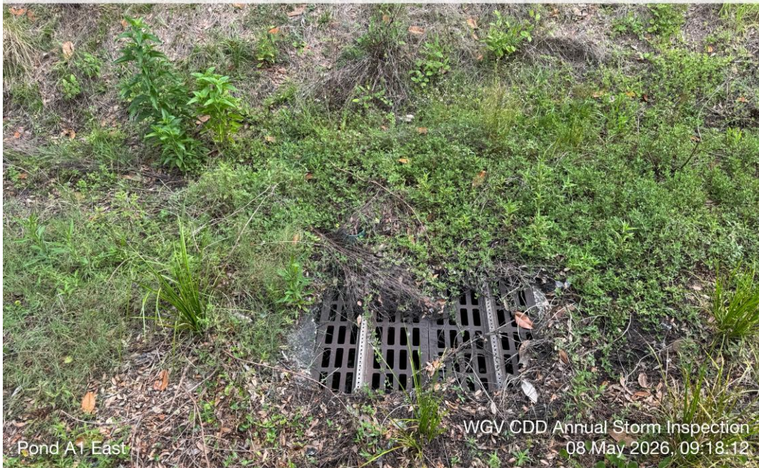
PHOTO #4.2 – Pond A1 East Bubble Up Structure #1 on May 8, 2026
