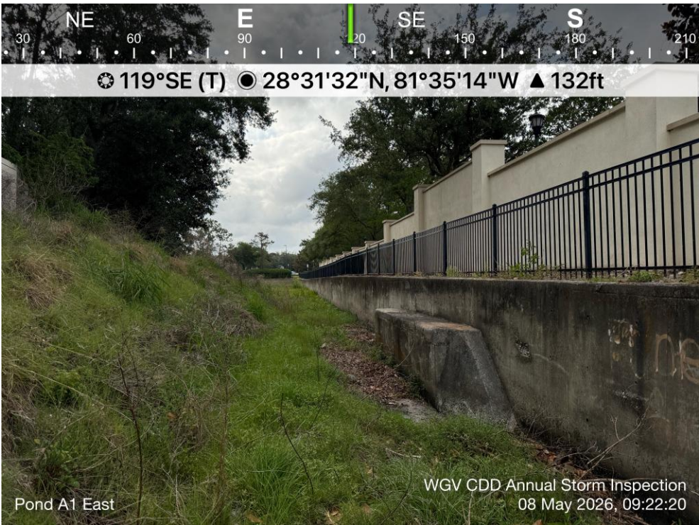
PHOTO #5.2 – Connection between Pond A1 East-West on May 8, 2026
