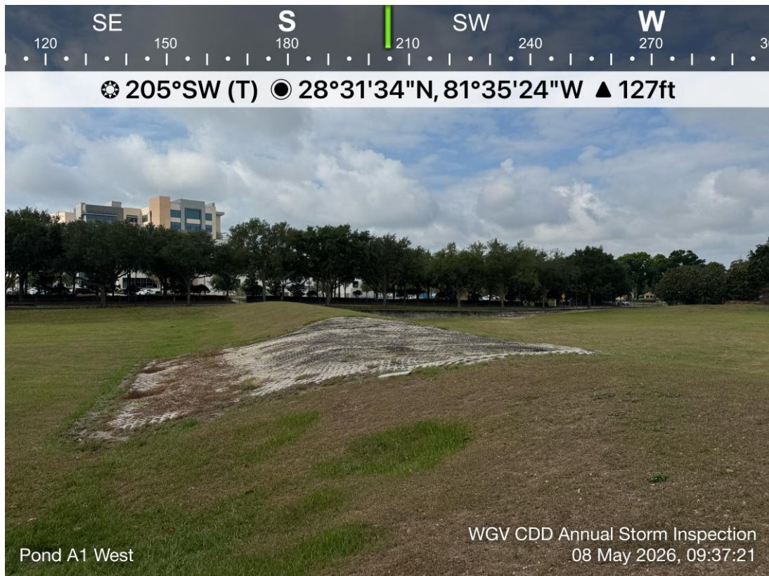
PHOTO #8.1 – Stabilized spillway from A1 West to A2 on May 8, 2026
