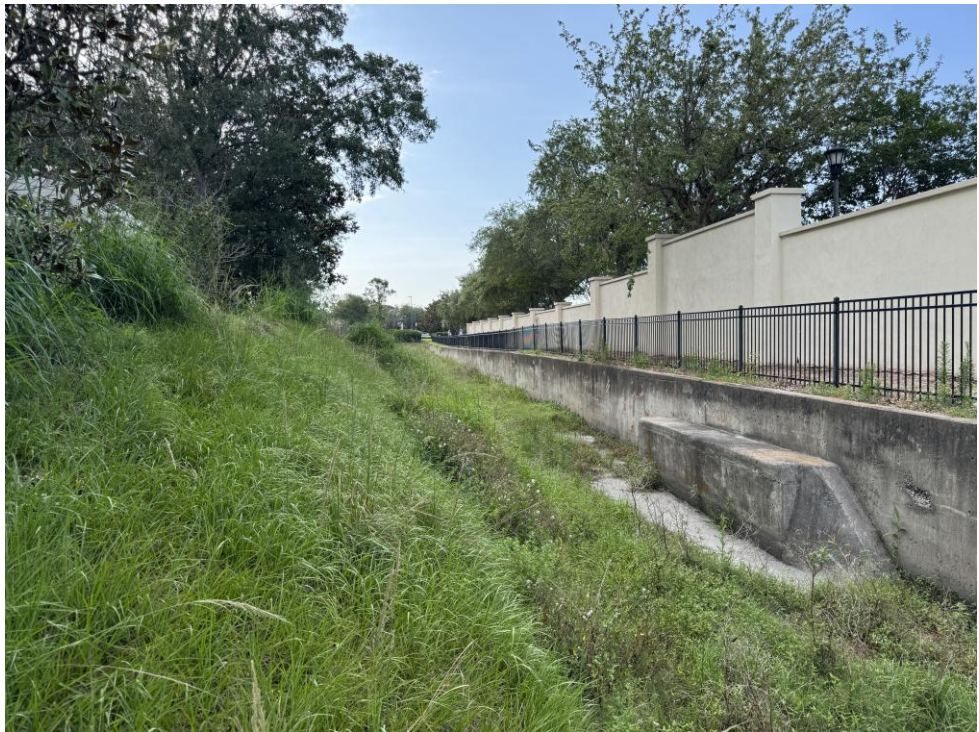
PHOTO #5.1 – Connection between Pond A1 East-West on May 23, 2025
