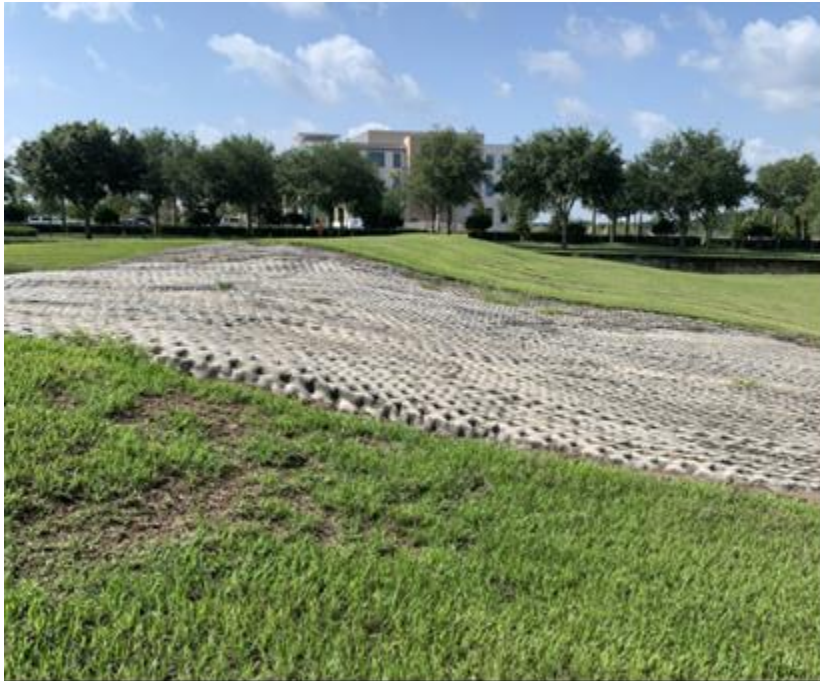
PHOTO #8 –Structural Weir from A1 to A2 on June 20, 2019
