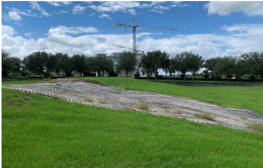
PHOTO #9 –Structural Weir from A1 to A2 on June 19, 2020
